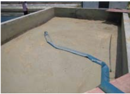
Cleaning the sand filter
