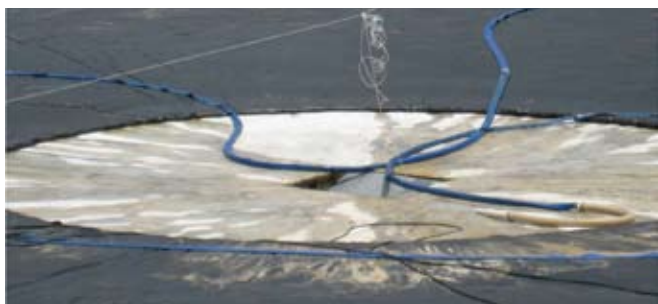
The waste is discharged from the middle of the pond
