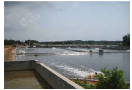
In the new model small culture ponds ranging from 3 to 5 mu (0.2-0.33 ha) are used
